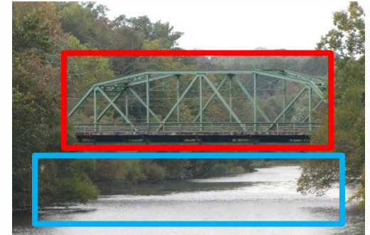
Iron bridge over the Duck river .
